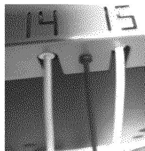
3. With the four security screws removed, the cable management bracket can be lifted out of place.
